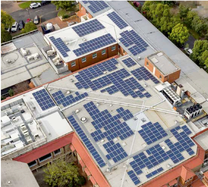
A bird's eye view of 500+ solar panels atop Burnside Hospital
